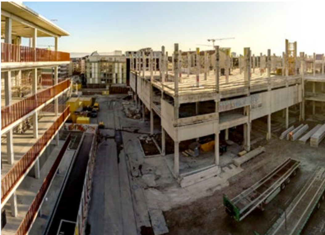
Rückbau Volta Nord Baufeld 4 © derek li wan po photography gmbh
